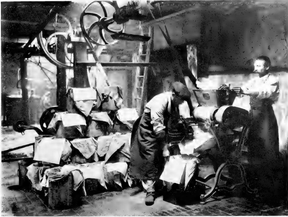
4—Kneading the Mass with a Roller-kneading Machine
